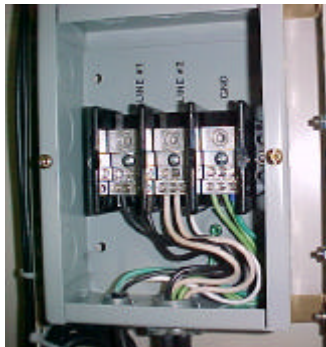
Figure 3-5: AC Input Box Assembly
