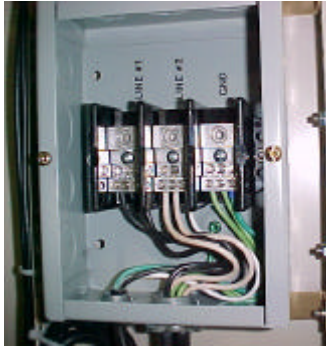
Figure 3-3: AC Input Box Assembly
