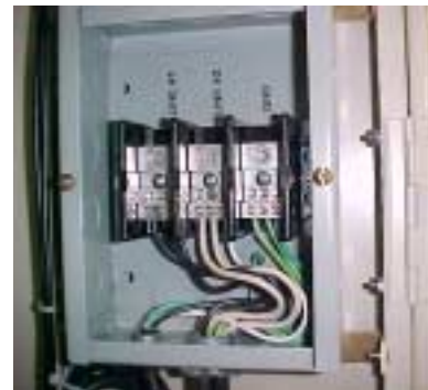
Figure 3-4. AC Input Box Assembly.
