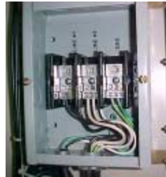
Figure 3-5: AC Input Box Assembly
