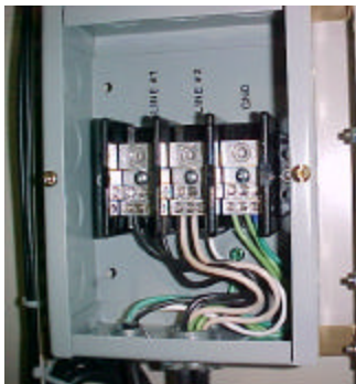
Figure 3-3: AC Input Box Assembly
