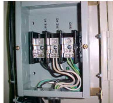
Figure 3-4. AC Input Box Assembly.
