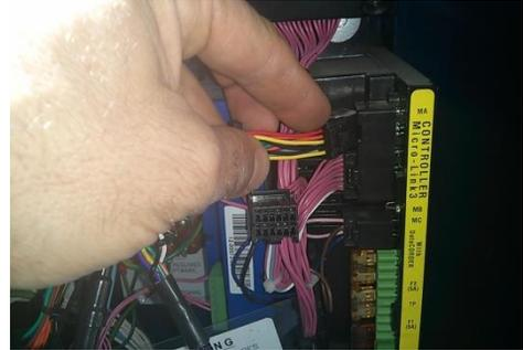
**3** Connect controller male connector to ArrowTrack female
