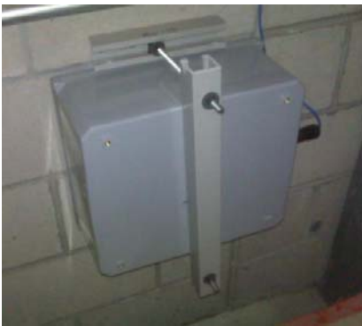
The sensor can be wall mounted as shown.
