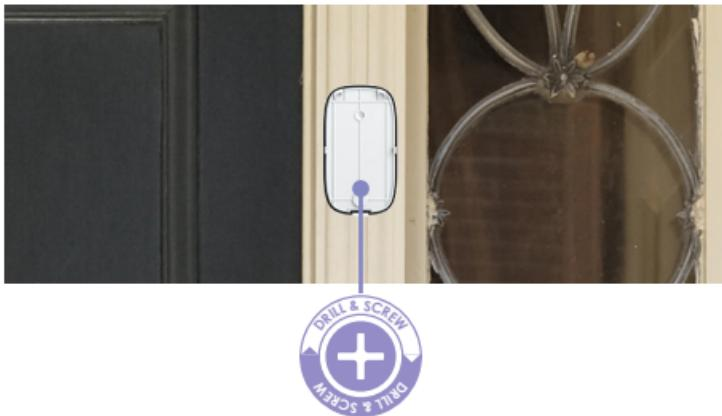
2. Place the backplate in position, mark and drill mounting holes, then screw into place.
