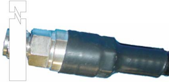
Figure 2-6 Apply Rubber Sealing Tape
