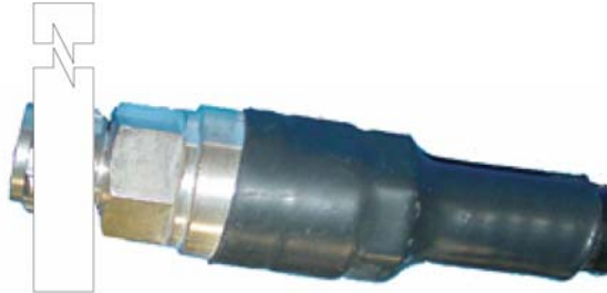
Figure 2-6 Apply Rubber Sealing Tape
