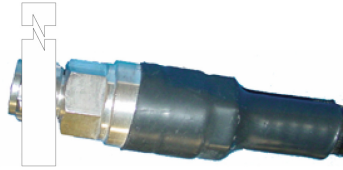
Figure 2-7 Apply Rubber Sealing Tape
