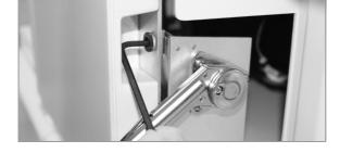
2 Locate the air relief valve to the right of the elevator door opening.
