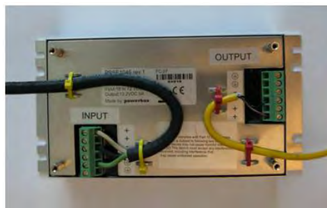
Figure 17: Cables Attached to the Power Supply
