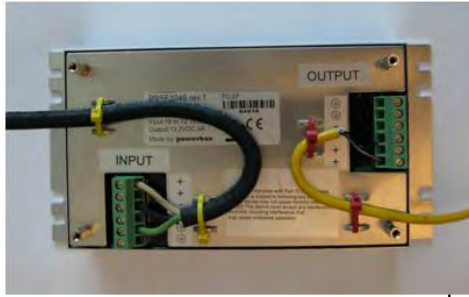
Figure 48: Cables Attached to the Power Supply
