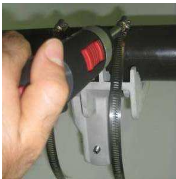
Figure 4.2 Using Special Hose Clamps & Screwing the Clamps
