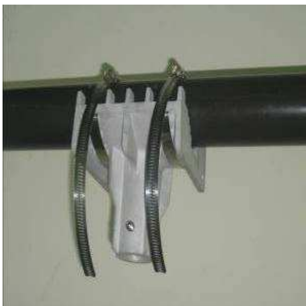
Figure 4.2 Using Special Hose Clamps & Screwing the Clamps
