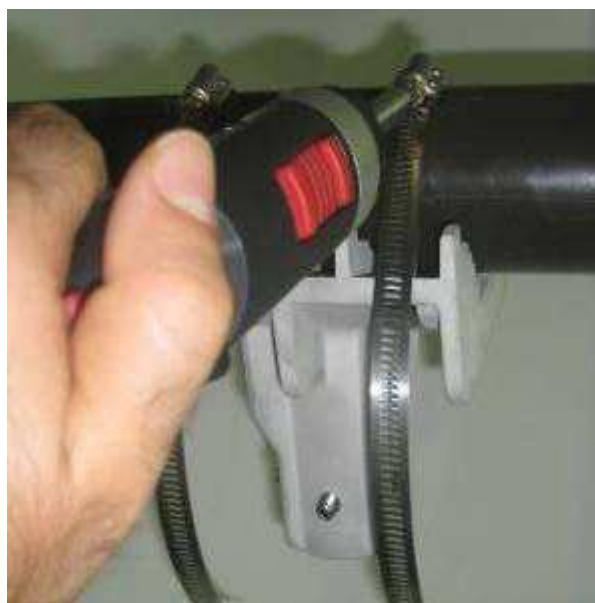
Figure 4.2 Using Special Hose Clamps & Screwing the Clamps
