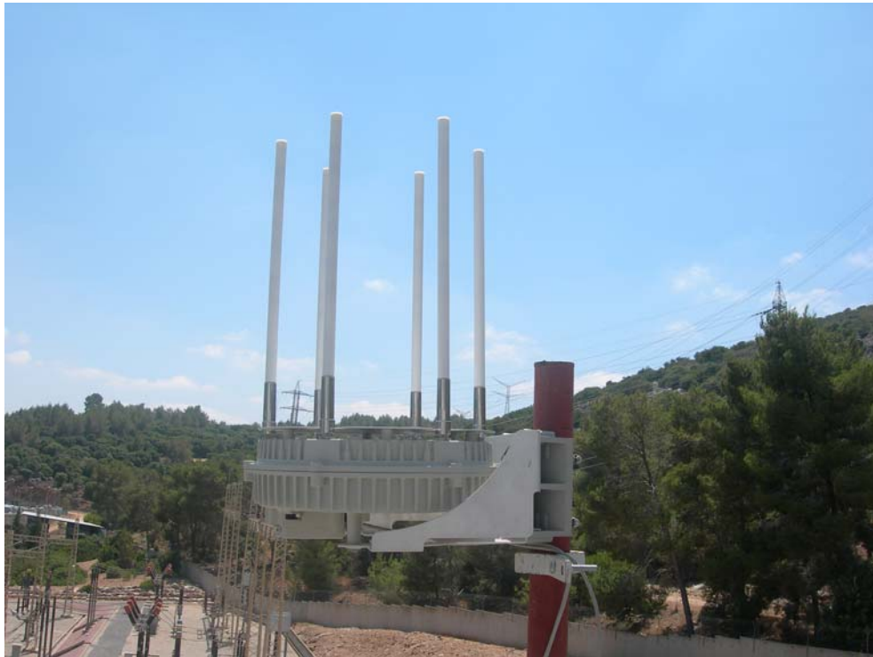
Figure 3.3. Mounting on a Pole
