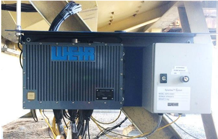
Figure 6-9 - MPM & PSU installed on mounting plate
