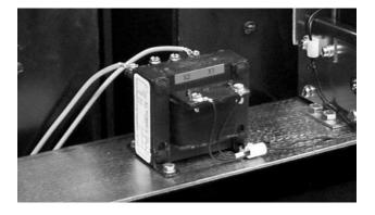
E. Attach the Glass Poly Insulation Plate to the top of the CPT, as shown, using the screws and lock washers supplied with the CPT kit.
