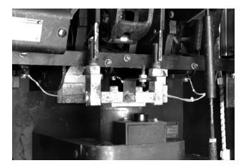
E. For Kits Supplied with a Breaker Mounted CPT Only. Route the Line Side HV Wires to the rear of the Breaker through the opening in the Breaker Back Plate and along the rear of the Breaker to the top Phase Frames.
