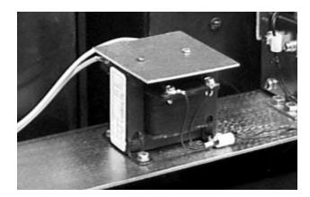
F. Attach the appropriate warning label for the Breaker to the left of the CPT on the Trip Unit Mounting Platform.
