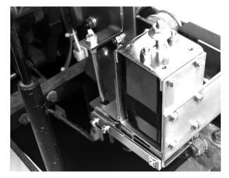
F. Connect a 24 VDC power supply to the DTA terminals; positive to positive and negative to negative. Close the Breaker manually. Energize the DTA to trip the Breaker; de-energize when the Breaker trips. Make certain that the DTA resets. If the Breaker fails to properly trip or reset, it may be necessary to shorten the brass spacer on the Reset Assembly Shaft. Make the necessary adjustments until the trips and resets are sure and positive each time.
