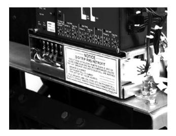
B. Route the Sensor Harness between the Glass Poly Insulation Barrier and the back of the Trip Unit, then down along the right Trip Unit Mounting Bracket and through the hole in the Breaker Back Plate as shown. Secure the Sensor Harness as shown using the wire clamps and (6) .138-20  $\times$  .500" thread cutting screws supplied.
