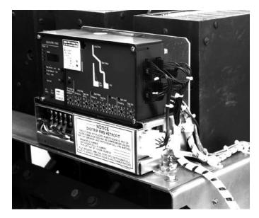
A. Feed the Sensor Harness through the hole in the left side of the Aux. CT Module. Connect the Sensor Harness to the proper terminals on the Aux. CT Module. Refer to Section 12 of the Retrofit Application Data, supplied with the Retrofit Kit, for detailed wiring specifications.
