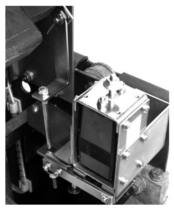
A. Mount the DTA Mounting Bracket to the right Breaker side panel, as shown, using the holes drilled in Step 5 A and the (2)  $.312-18 \times .750"$ screws, (2) flat washers, (2) lock washers, and (2) nuts provided.
