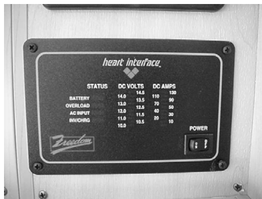
Inverter/Charger Remote Panel
