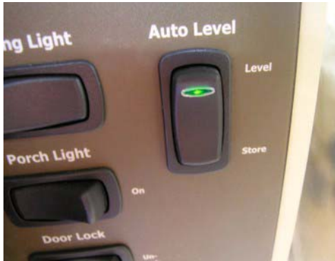
Auto Level Switch inside Entrance Door
