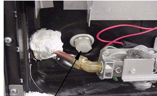
Water Heater Drain Plug Remove with socket
