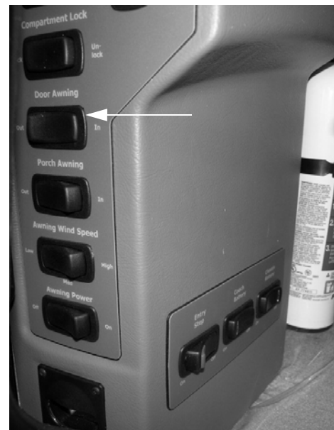
Over the Door Awning Switch - Typical View (Located near the entrance door)
