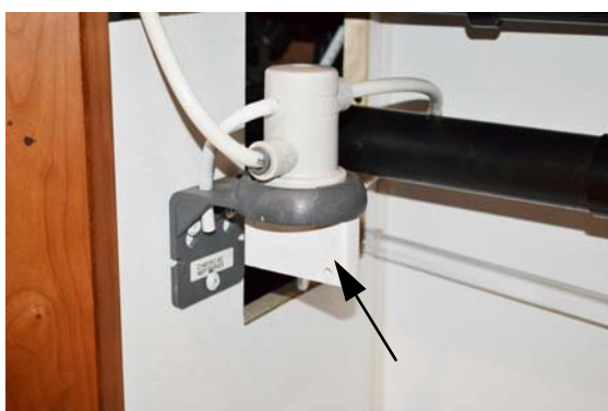
Diverter Plug (installed in filter socket)
