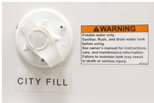
Fresh (City) Water Inlet -Typical View
