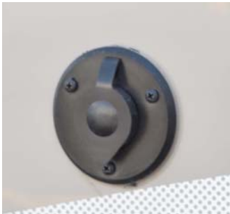
Exterior TV Connection (Located near entrance door) -Typical View
