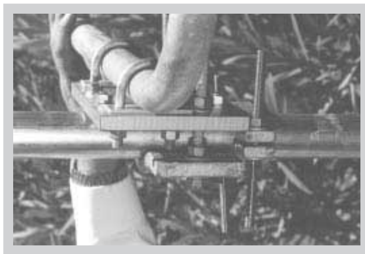
Figure 4.21 - Azimuth Adjustment Clamp Assembly
