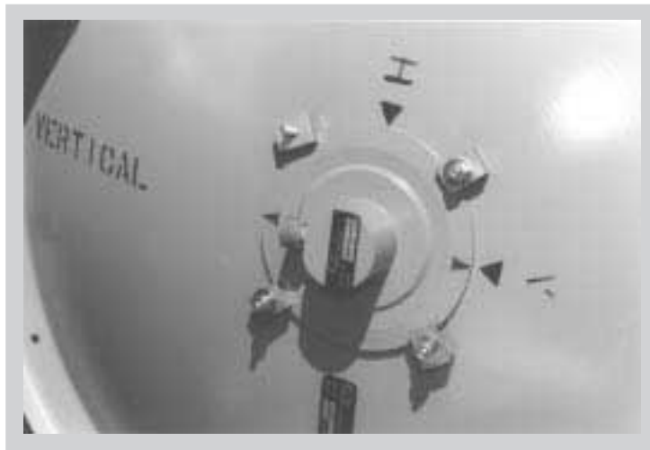
Figure 4.19 - Feed Horn Installation for Vertical Polarized Operation
