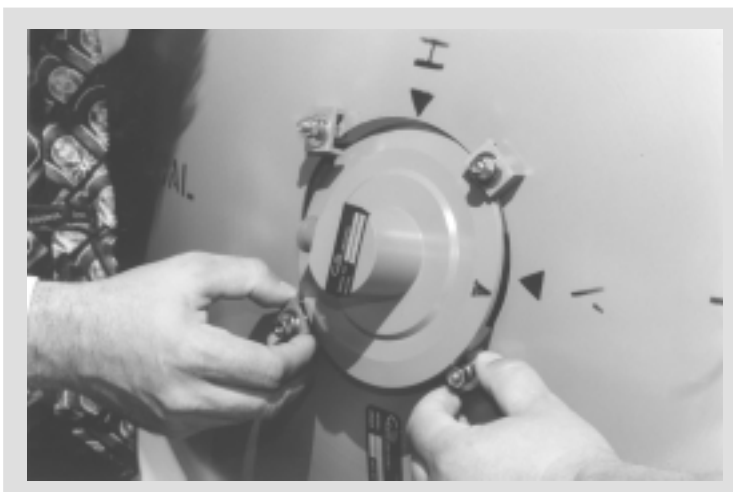
Figure B.13 - Feed Horn Installation
