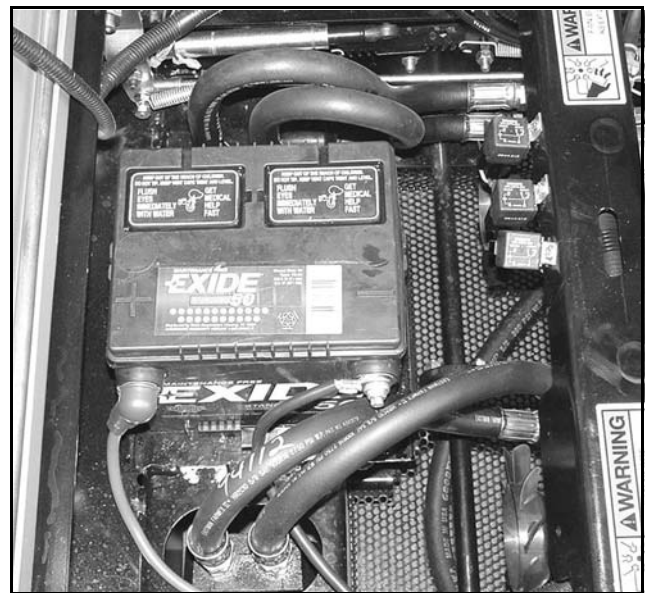
Figure 9. Battery Located under Seat
