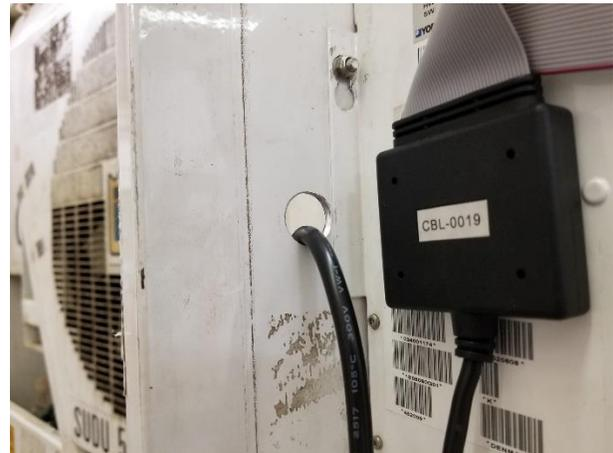
Figure 2: Size of hole – 19mm
