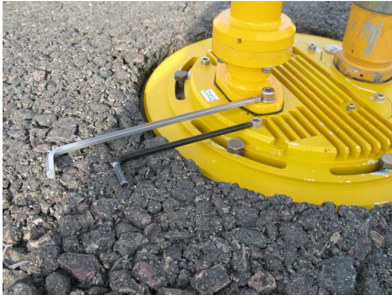
Figure 3: M6 and M8 wrenches for fastening upper and lower unit screws
