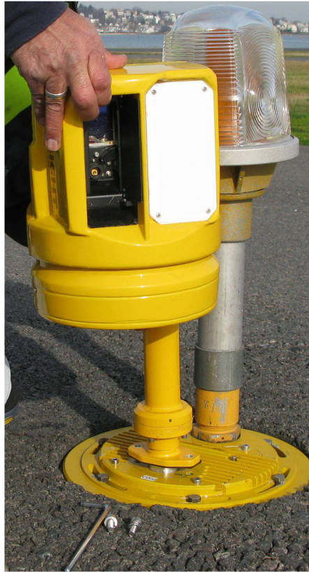
Figure 26: Upper unit installation
