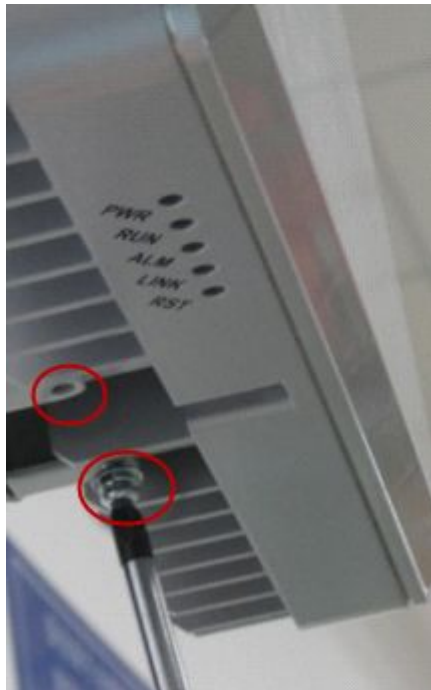
Figure 6-13 Fixing the ZXSDR BS8802 C100
