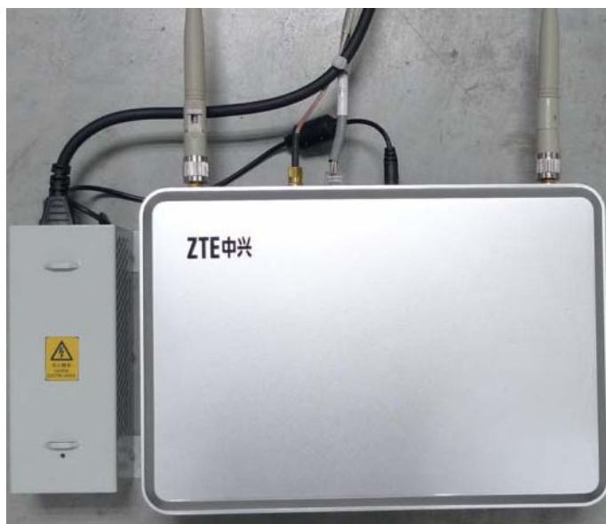
Figure 6-10 Separately Wall-Mounted ZXSDR BS8802 C100 and Power Adapter
