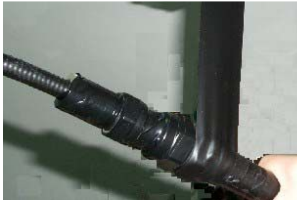
FIGURE 131 WATERPROOF INSULATION ADHESIVE TAPE WRAP
