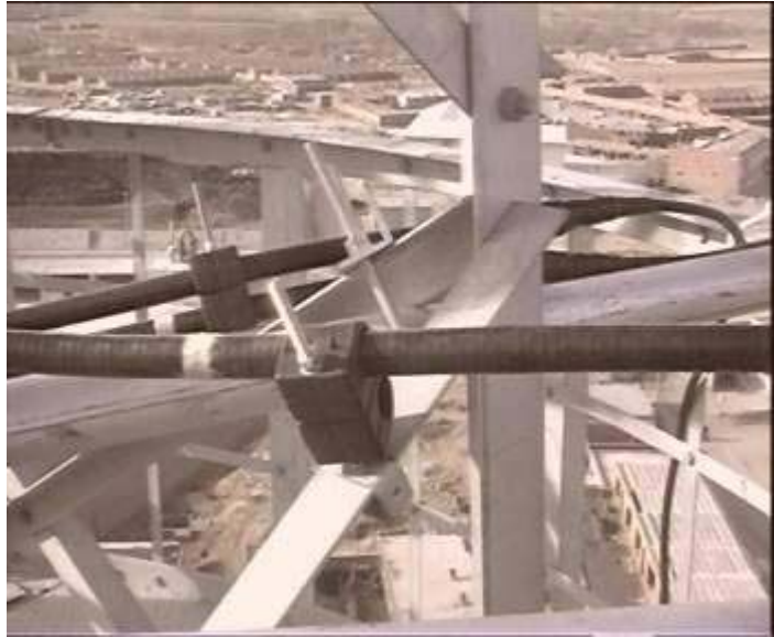
FIGURE 118 FEEDER FIXATION ON THE TOWER (ONE KIT AND TWO FIXATION CLIPS)
