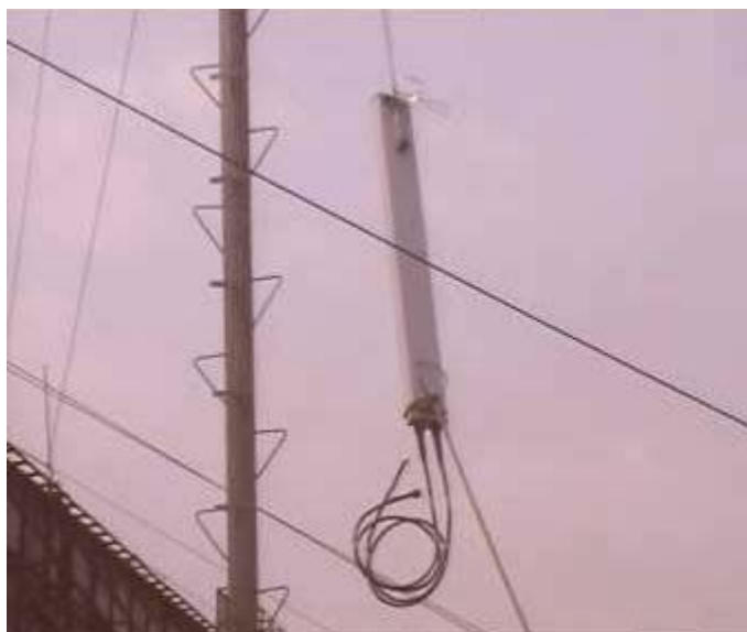
FIGURE 73 HOISTING ANTENNA
