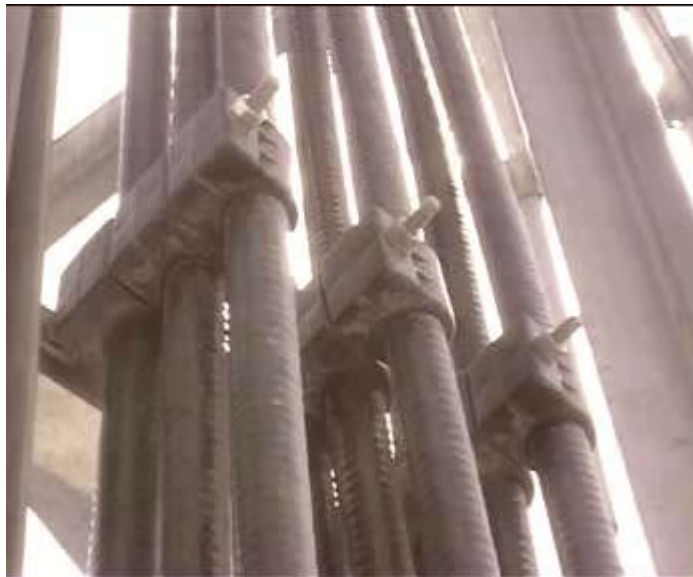
FIGURE 119 FEEDER FIXATION ON THE TOWER (ONE KIT AND THREE FIXATION CLIPS)
