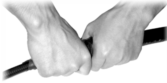
Fig. 10.6-3 Wrapping the Waterproof Adhesive Tapes (3)
