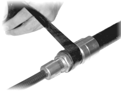
Fig. 10.6-1 Wrapping the Waterproof Adhesive Tapes (1)
