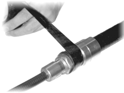
Fig. 10.6-1 Wrap the Waterproof Adhesive Tapes (1)
