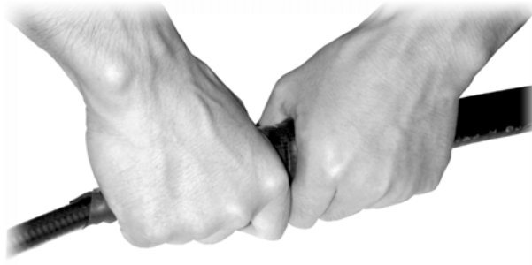
Fig. 10.6-3 Wrap the Waterproof Adhesive Tapes (3)
