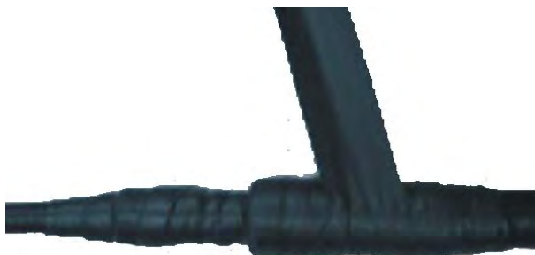
Figure 5-28 Wrapping Three Layers of Water Insulating Tape (the Third Layer)
