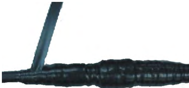
Figure 5-30 Wrapping Three Layers of PVC Insulating Tape (the Second Layer)
