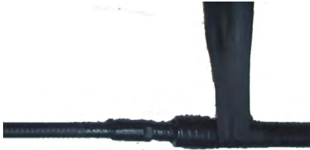
Figure 5-26 Wrapping Three Layers of Water Insulating Tape (the First Layer)
