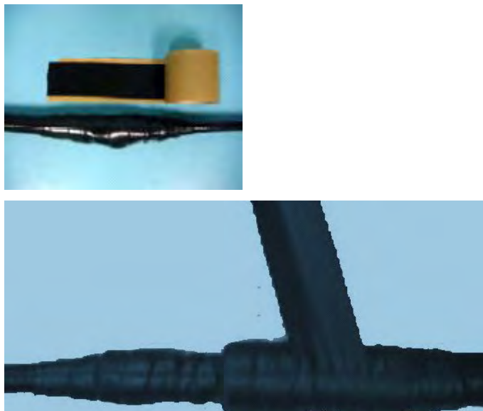
Figure 4-4 Wrapping Three Layer of Plaster
