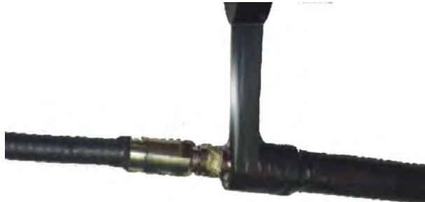
Figure 5-25 Wrapping a Layer of PVC Insulating Tape
