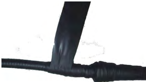
Figure 5-27 Wrapping Three Layers of Water Insulating Tape (the Second Layer)
