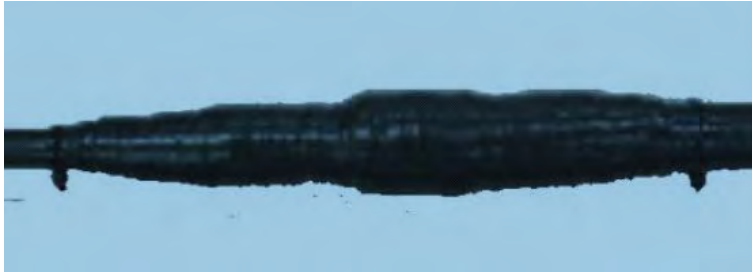
Figure 4-6 Binding Cable Fasteners
