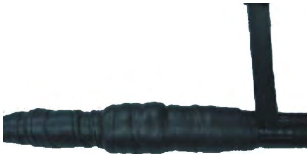
Figure 5-29 Wrapping Three Layers of PVC Insulating Tape (the First Layer)
