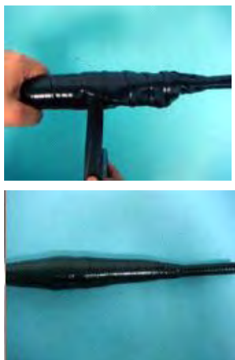
Figure 4-5 Wrapping a Layer of Tape
