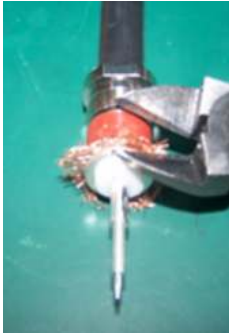
FIGURE 99 - CUTTING SHIELDED LAYER
