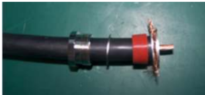
FIGURE 96 - AFTER STRIPPING INSULATION LAYER
