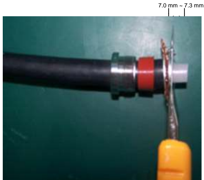
FIGURE 95 - STRIPPING INSULATION LAYER
