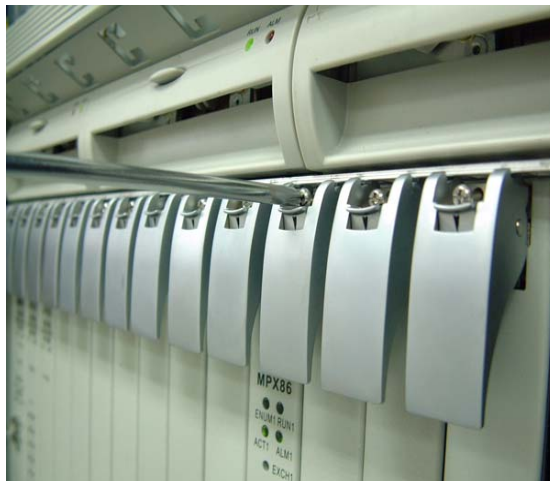
FIGURE 85 - BOARD PLUGGING (STEP 3)
