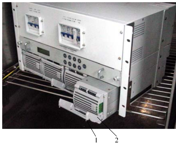
FIGURE 18 - TAKING OUT RECTIFIER MODULE
