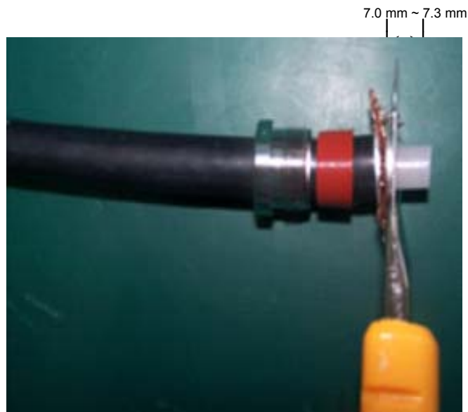
FIGURE 74 - STRIPPING INSULATION LAYER
