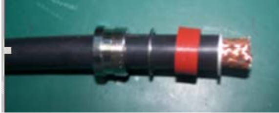
FIGURE 71 - EXTERNAL CONDUCTOR ASSEMBLY
