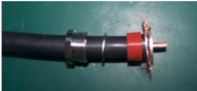
FIGURE 75 - AFTER STRIPPING INSULATION LAYER
