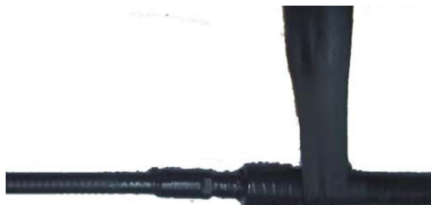
FIGURE 95 WRAPPING THREE LAYERS OF WATER INSULATING TAPE (THE FIRST LAYER)
