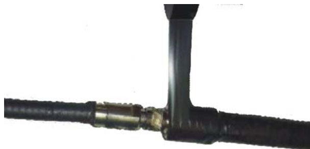
FIGURE 94 WRAPPING A LAYER OF PVC INSULATING TAPE
