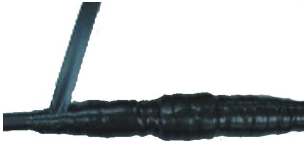
FIGURE 99 WRAPPING THREE LAYERS OF PVC INSULATING TAPE (THE SECOND LAYER)
