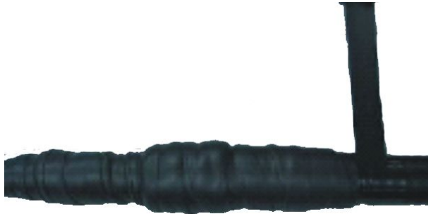
FIGURE 98 WRAPPING THREE LAYERS OF PVC INSULATING TAPE (THE FIRST LAYER)
