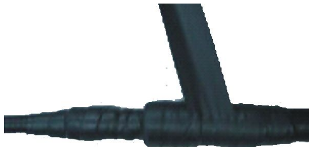
FIGURE 97 WRAPPING THREE LAYERS OF WATER INSULATING TAPE (THE THIRD LAYER)
