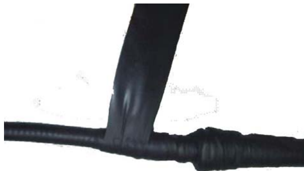
FIGURE 96 WRAPPING THREE LAYERS OF WATER INSULATING TAPE (THE SECOND LAYER)
