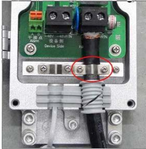
Figure 3-38 PIMDC Connection (to Lightning Protection Box)
