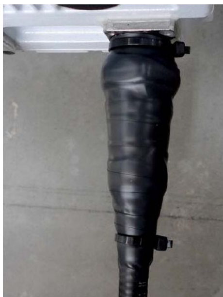
Figure A-4 Fixing Both Ends
