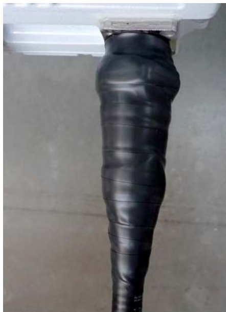
Figure A-3 Wrap Three Layers of UV Resistance Tape
