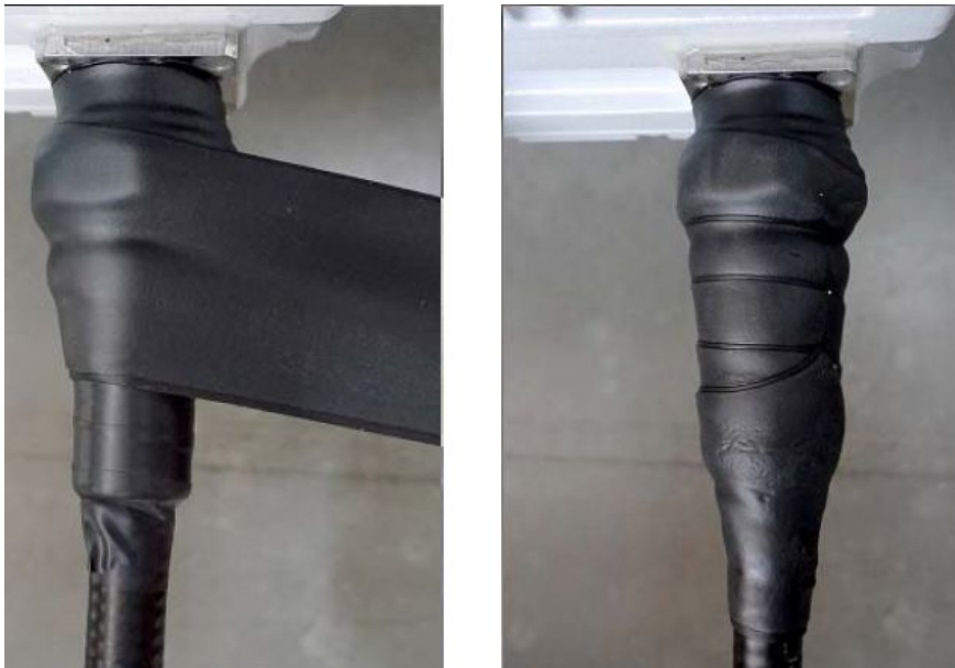
Figure A-2 Wrapping Three Layers of Waterproof Tape
