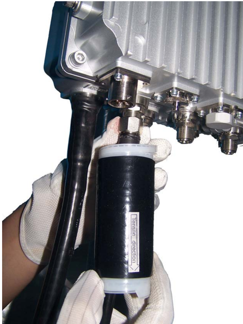
FIGURE 90 SCREWING DOWN FEEDER CONNECTOR
