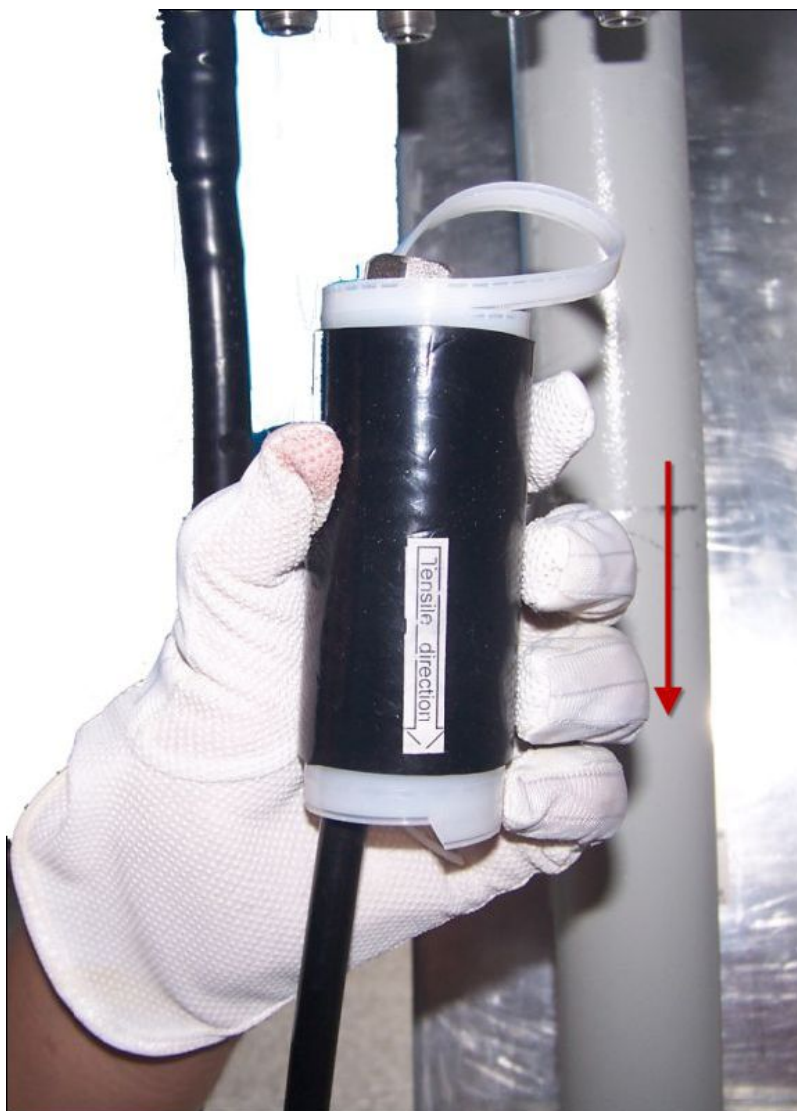
FIGURE 89 FEEDER THROUGH SHRINKABLE SLEEVE
