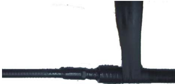
FIGURE 60 WRAPPING THREE LAYERS OF WATER INSULATING TAPE (THE FIRST LAYER)
