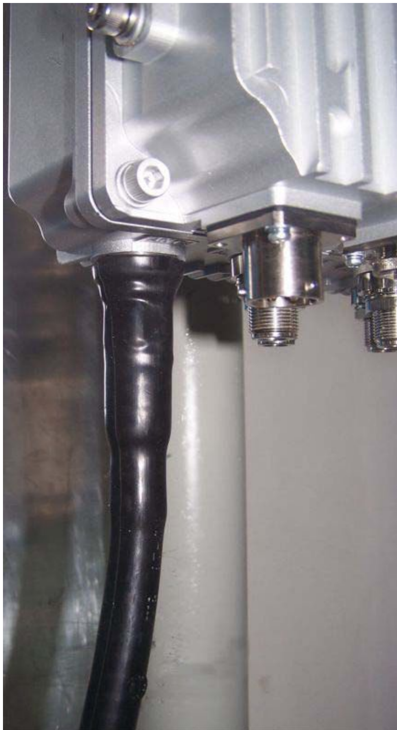
FIGURE 94 COMPLETING WATERPROOF PROCESSING
