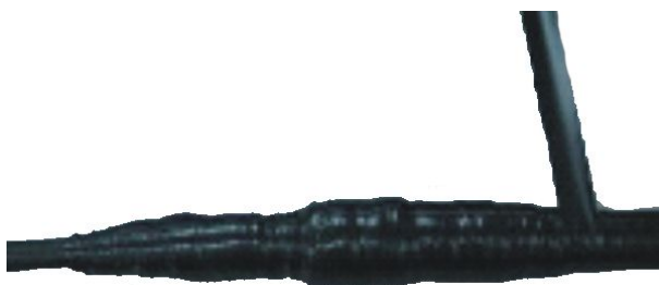
FIGURE 65 WRAPPING THREE LAYERS OF PVC INSULATING TAPE (THE THIRD LAYER)
