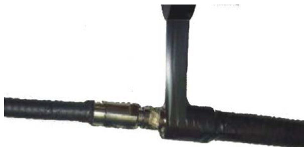
FIGURE 59 WRAPPING A LAYER OF PVC INSULATING TAPE
