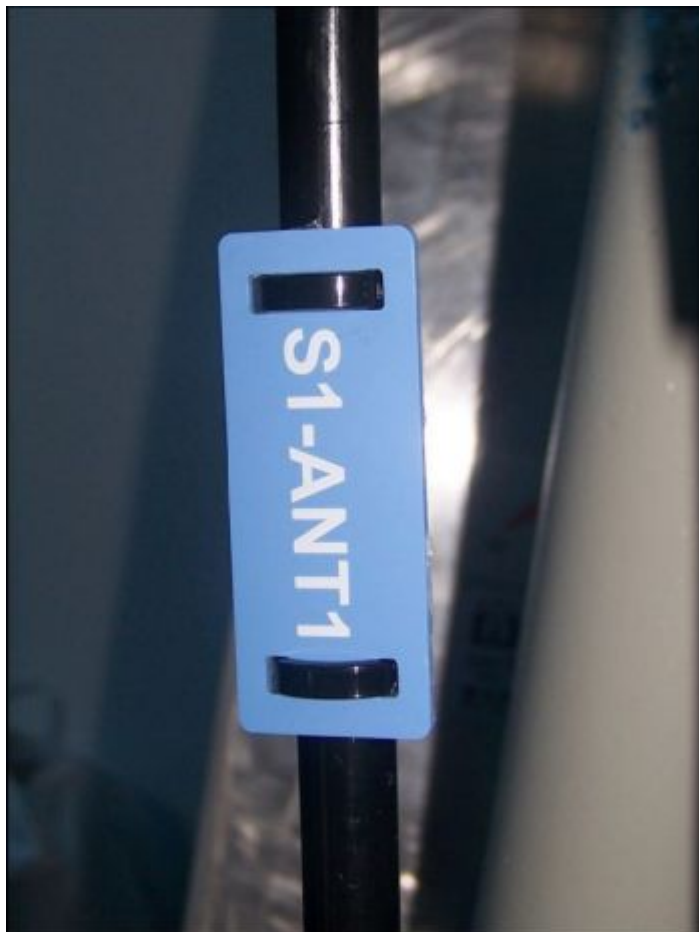
FIGURE 54 BINDING FEEDER LABEL
