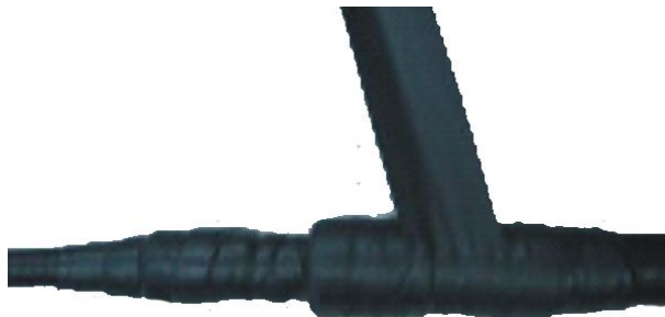
FIGURE 62 WRAPPING THREE LAYERS OF WATER INSULATING TAPE (THE THIRD LAYER)
