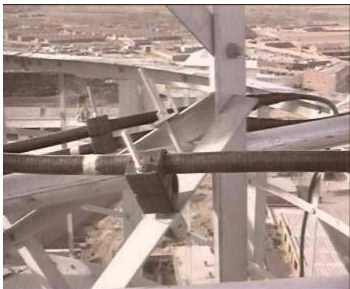
FIGURE 86 FEEDER FIXATION ON TOWER (TWO-COMBINED FEEDER CLIP)
