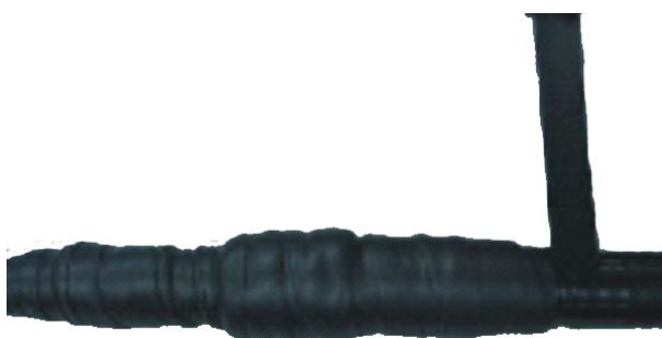
FIGURE 63 WRAPPING THREE LAYERS OF PVC INSULATING TAPE (THE FIRST LAYER)
