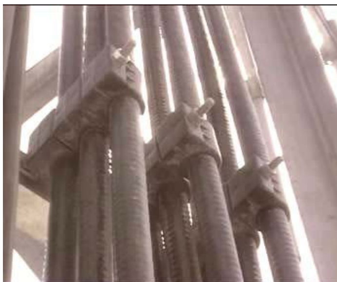
FIGURE 87 FEEDER FIXATION ON TOWER (THREE-COMBINATION FEEDER CLIP)
