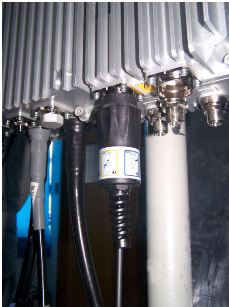
FIGURE 50 FASTENING THE SEALING GLAND
