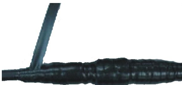
FIGURE 64 WRAPPING THREE LAYERS OF PVC INSULATING TAPE (THE SECOND LAYER)
