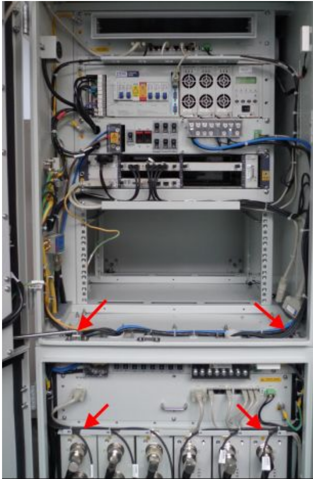
Figure 5-14 SFP Cable Layout
