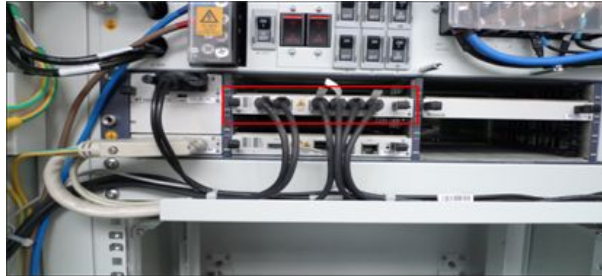
FIGURE 19 FS BOARD CONNECTING TO THE BBU
