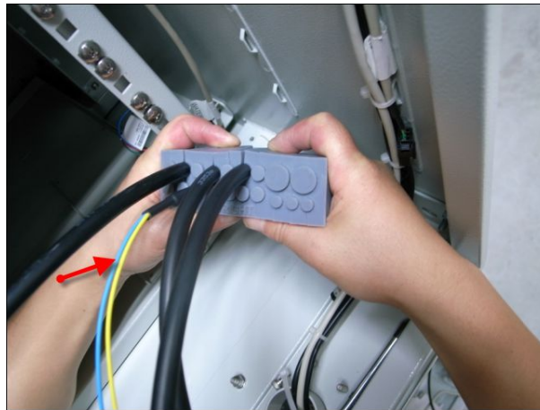
FIGURE 15 WATERPROOF MODULE THROUGH WHICH OPTICAL FIBERS PASS
