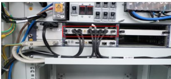
Figure 5-15 FS Board Connecting to the BBU
