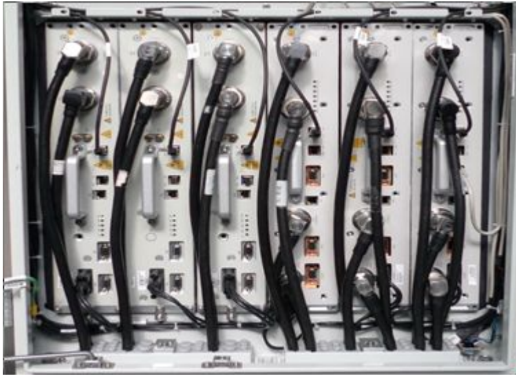
Figure 5-16 Antenna Feeder Jumper Installed Completely
