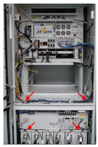
4. Insert SFP cables into the interfaces TX0RX0 to TX5RX5 of the BBU FS board according to the markings 0-5, as shown in Figure 5-15.
