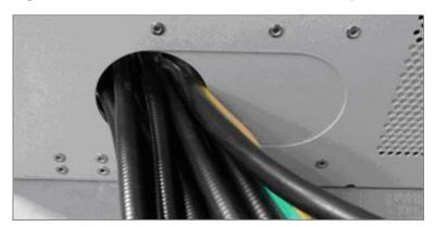
Figure 5-17 Lead-Out of the Antenna Feeder Jumper
