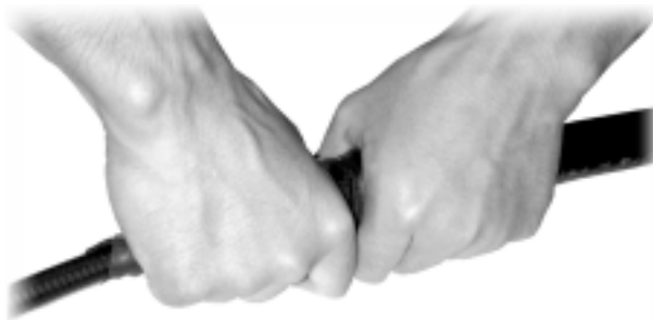
Fig. 8.6-12 Schematic Diagram of Wrapping Waterproof Adhesive Tape (3)
