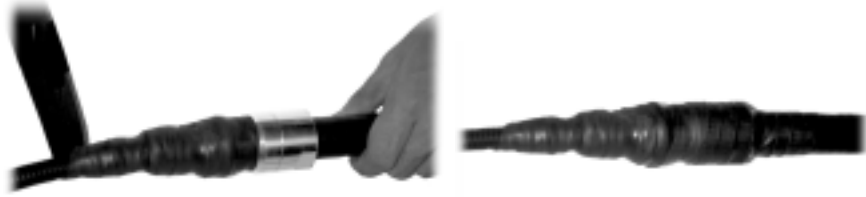
Fig. 8.6-11 Schematic Diagram of Wrapping Waterproof Adhesive Tape (2)
