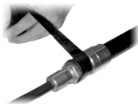
Fig. 8.6-10 Schematic Diagram of Wrapping Waterproof Adhesive Tape (1)
