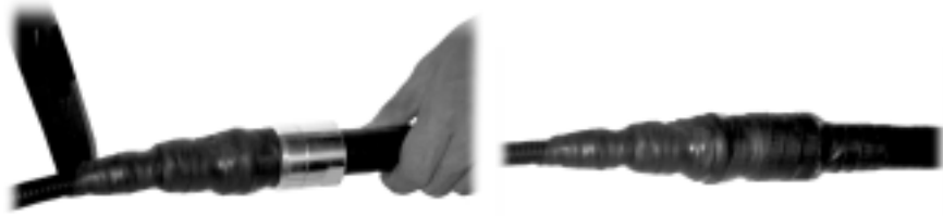
Fig. 8.6-11 Schematic Diagram of Wrapping Waterproof Adhesive Tape (2)
