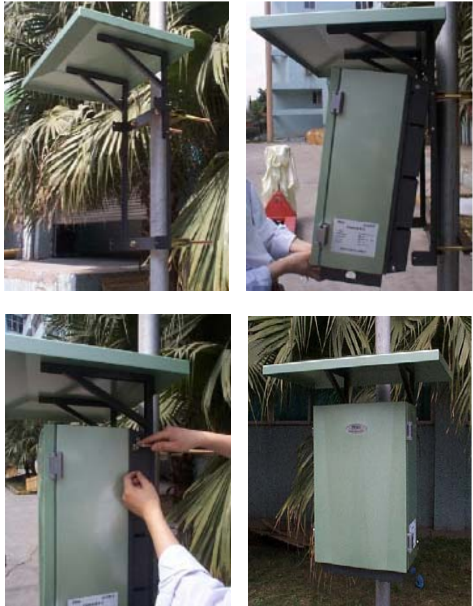
Fig. 4.2-4 Schematic Diagram of the Cabinet Fastened onto the Pole
