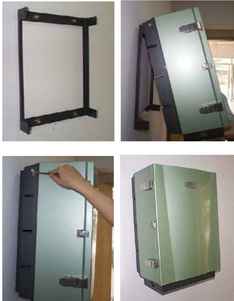
Fig. 4.2-6 Schematic Diagram of Installing the Cabinet onto the Wall
