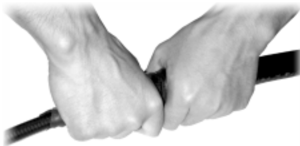
Fig. 8.6-12 Schematic Diagram of Wrapping Waterproof Adhesive Tape (3)
